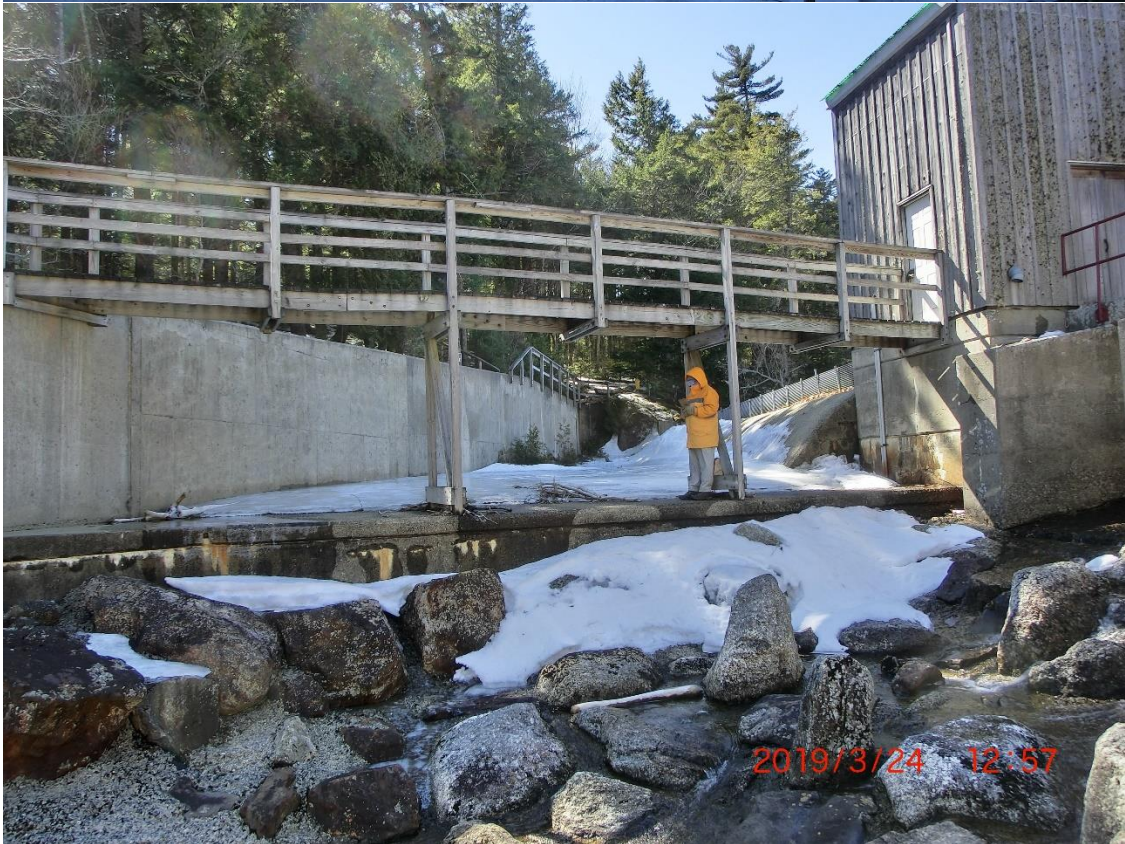
Photo 2-3 Spillway and Flume
