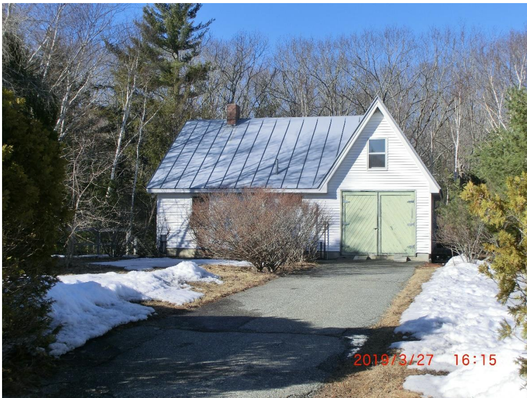
Photo 2-7 Powerhouse from Driveway
