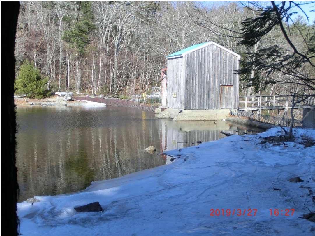
Photo 2-2 Green Lake Dam from the Southwest
