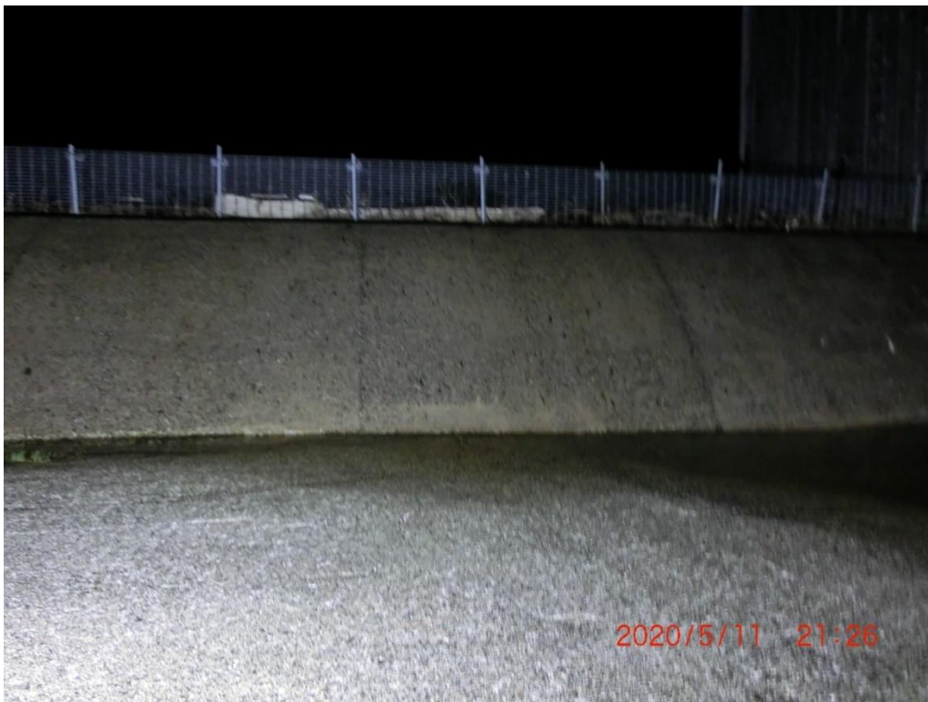
Photo 7-8 – Looking for eels at night – spillway
