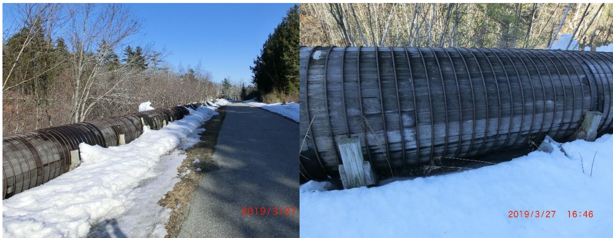
Photo 2-6 Wood Stave Penstock
