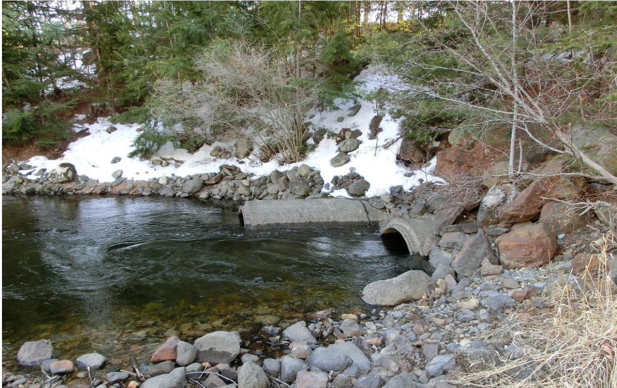
Photo 2-13 Tailwater Concrete Pipes
