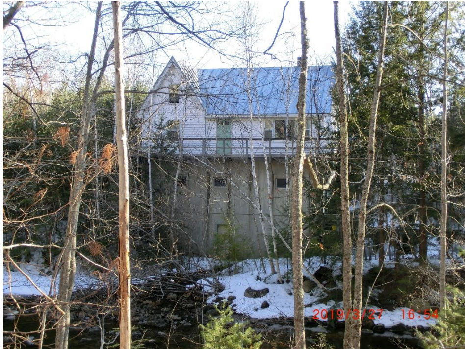
Photo 2-8 Powerhouse North Side
