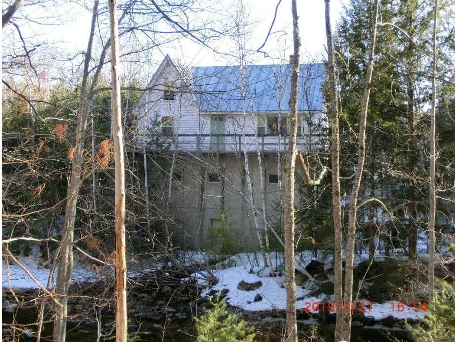
PHOTO 4-10 MAIN GENERATOR AND TURBINE
