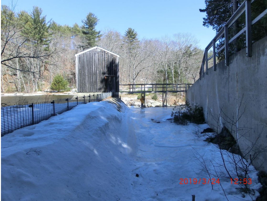
PHOTO 4-4 SPILLWAY AND FLUME
