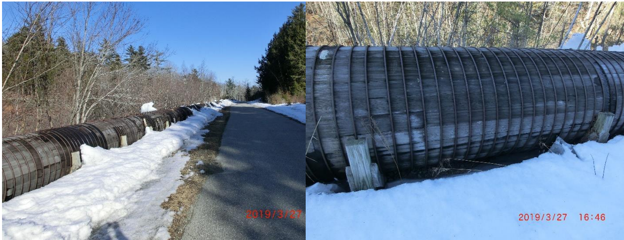
PHOTO 4-7 WOOD STAVE PENSTOCK
