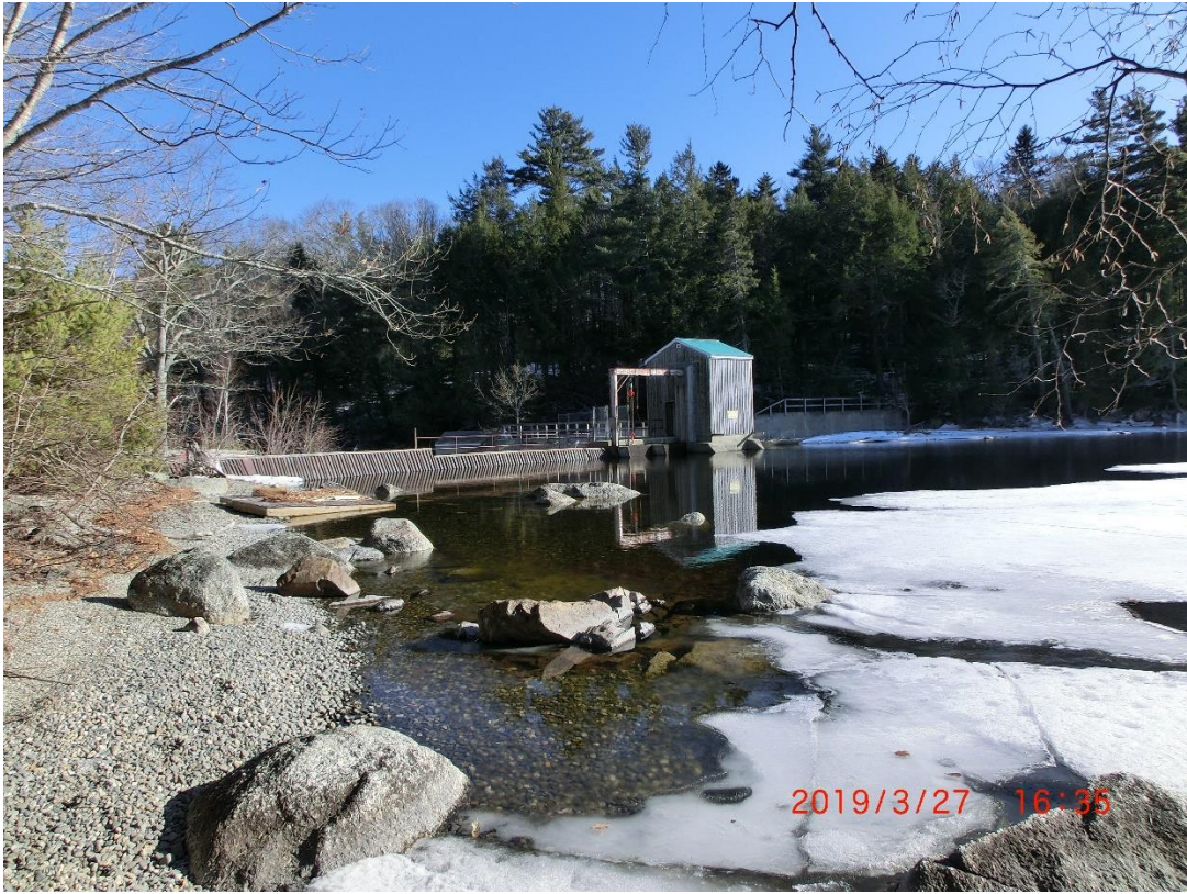
Photo 2-1 Green Lake Dam from the Northwest
