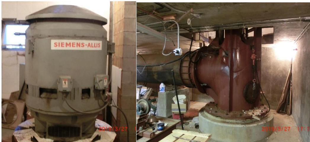
Photo 2-9 Main generator and turbine
