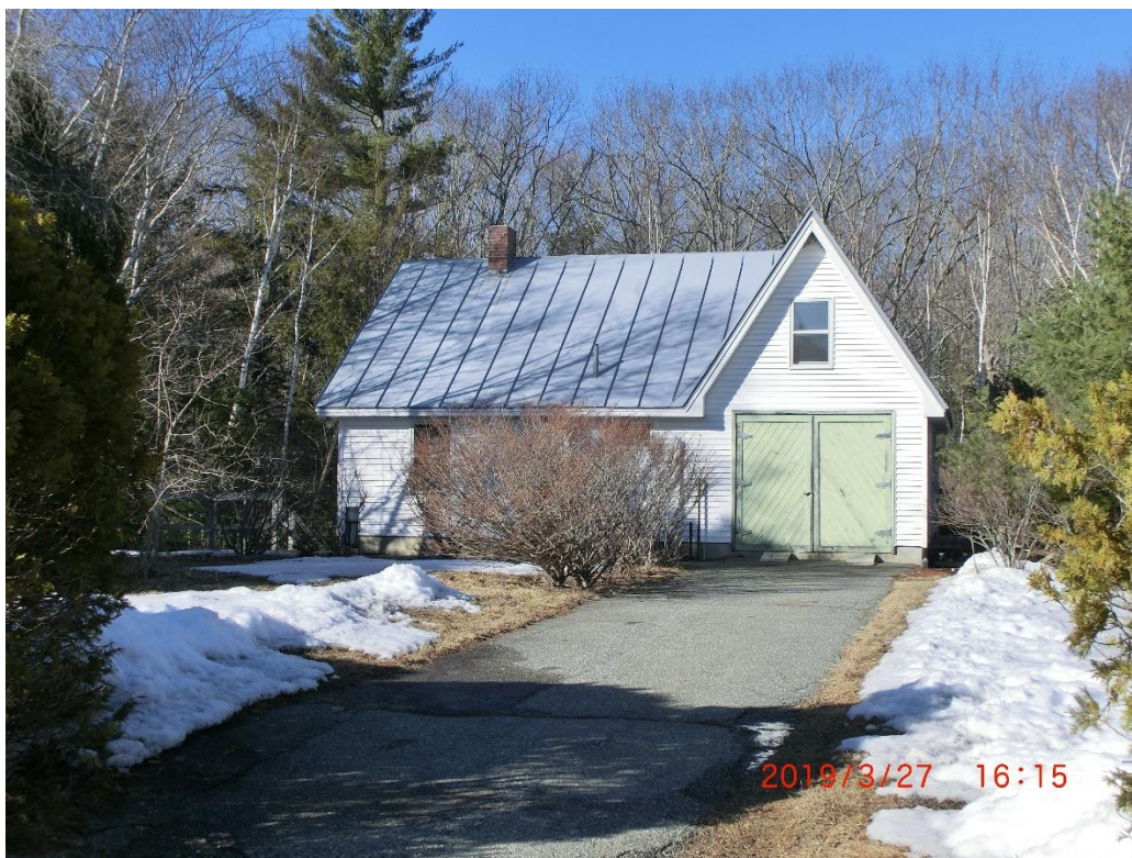
Photo 2-7 Powerhouse from Drive
