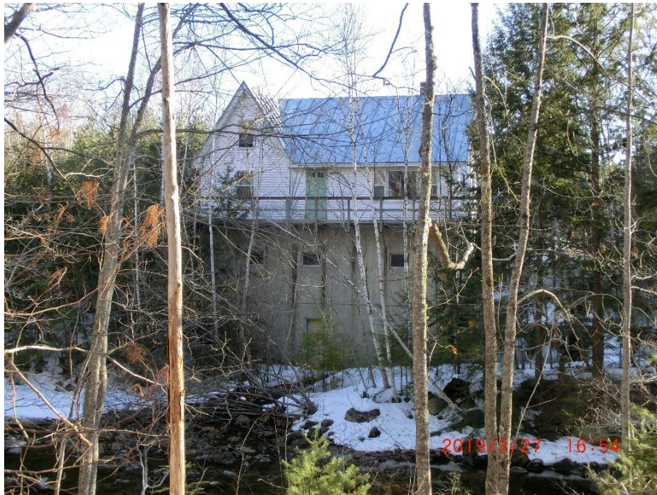
Photo 2-8 Powerhouse North Side
