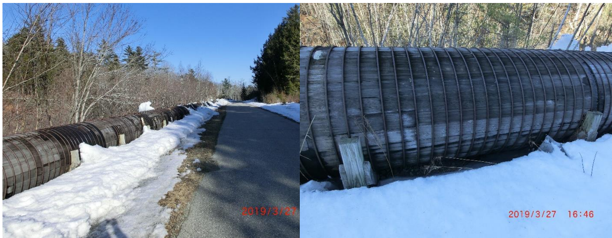
Photo 2-6 Wood Stave Penstock
