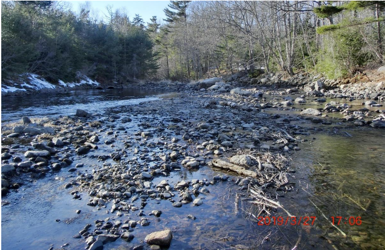
Photo 2-12 Reeds Brook Below Powerhouse, Tailwater on Left
